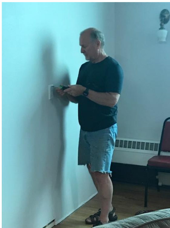
Max Davidson is seen putting the finishing touches on the new wall in the overflow room after taping, texturing and wiring.
